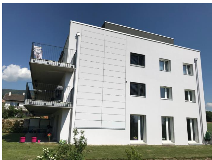
Left image: First realisation on an existing building with PV modules using Solaxess white films (Boudry, Switzerland).
